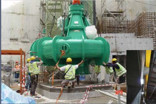
Setting first of ten 72,975-gpm pumps in the IPS
