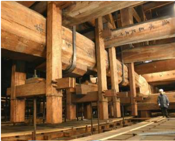
Wooden Structural System in Roof
