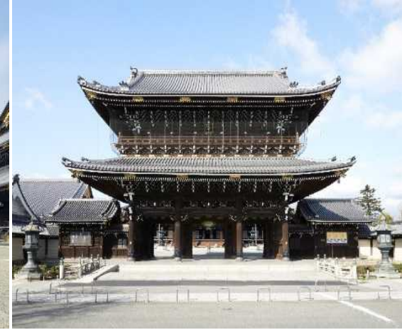
Renovation Completed Gate
