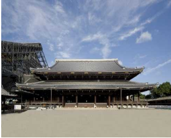
Renovation Completed Founder's Hall
