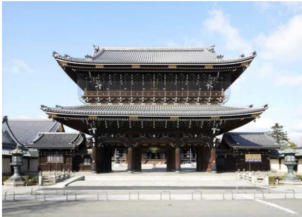
Founder's Hall Gate after renovation
