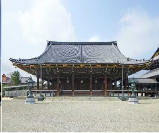
Renovation Completed Amida Hall
