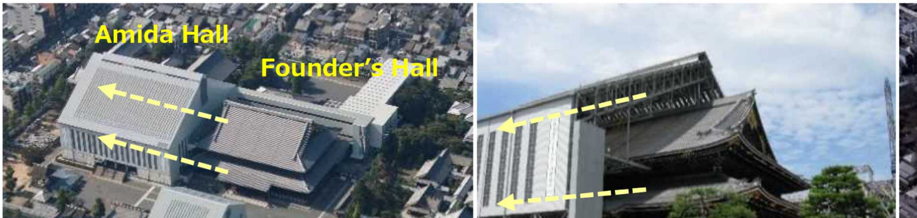
Sliding the Temporary Roof Structure
