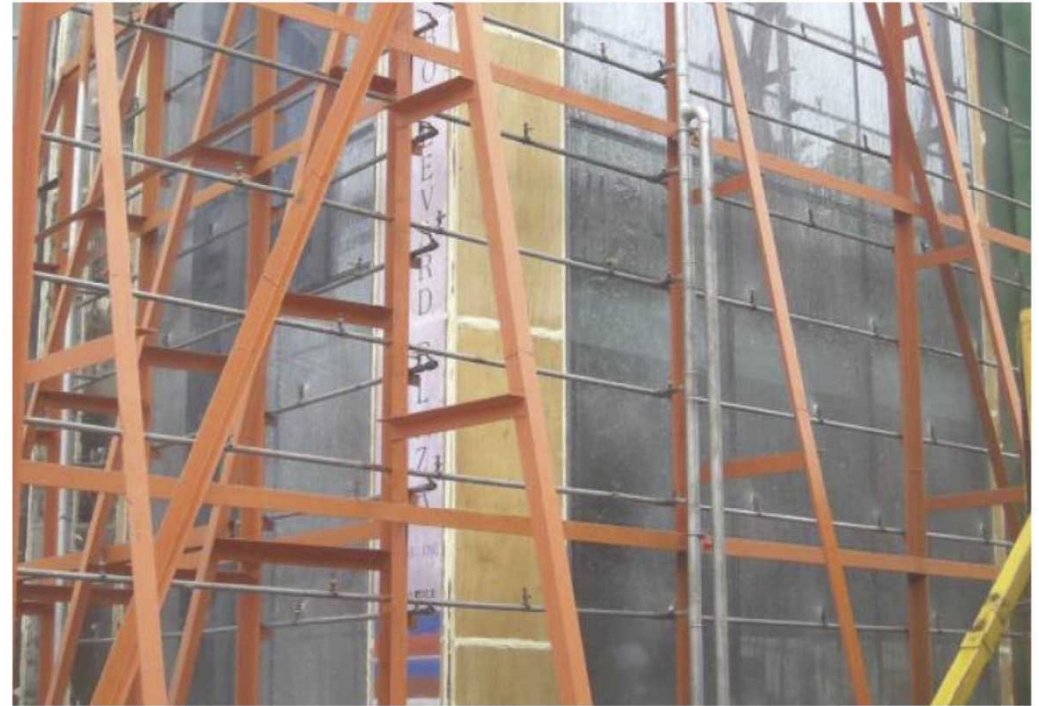
Curtain wall waterproofing test
