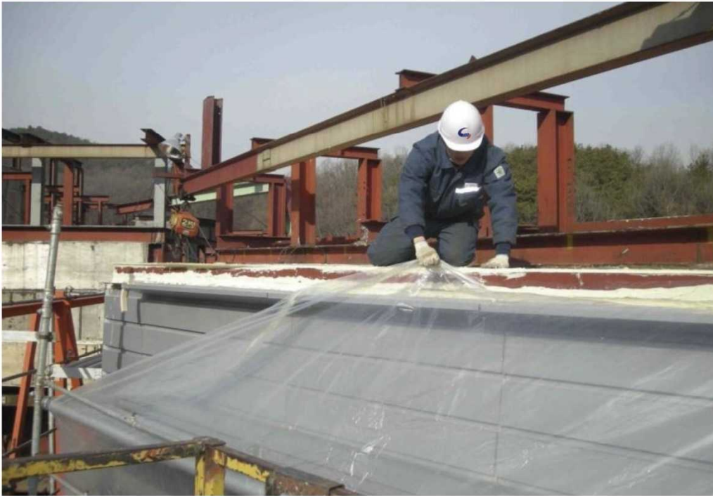
Curtain wall wind test
