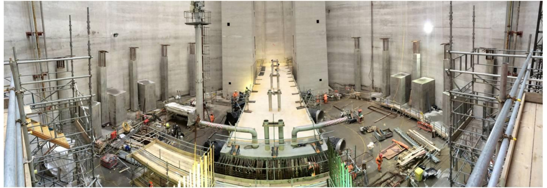
Pumping Station Bottom with Suction Tunnel Intake
