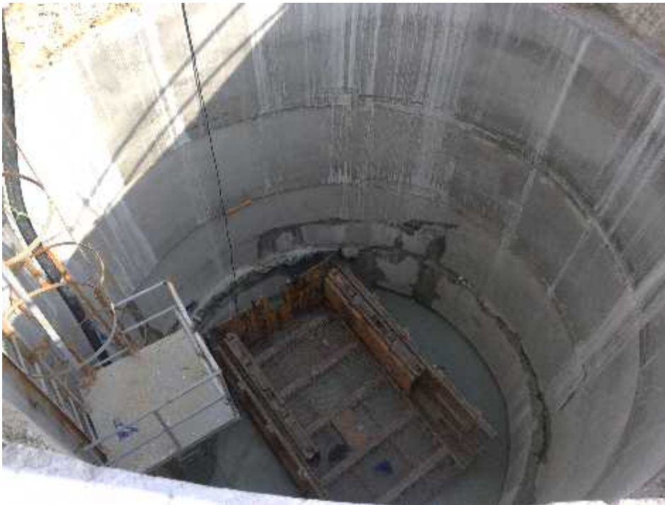
MTBM Launch Frame
