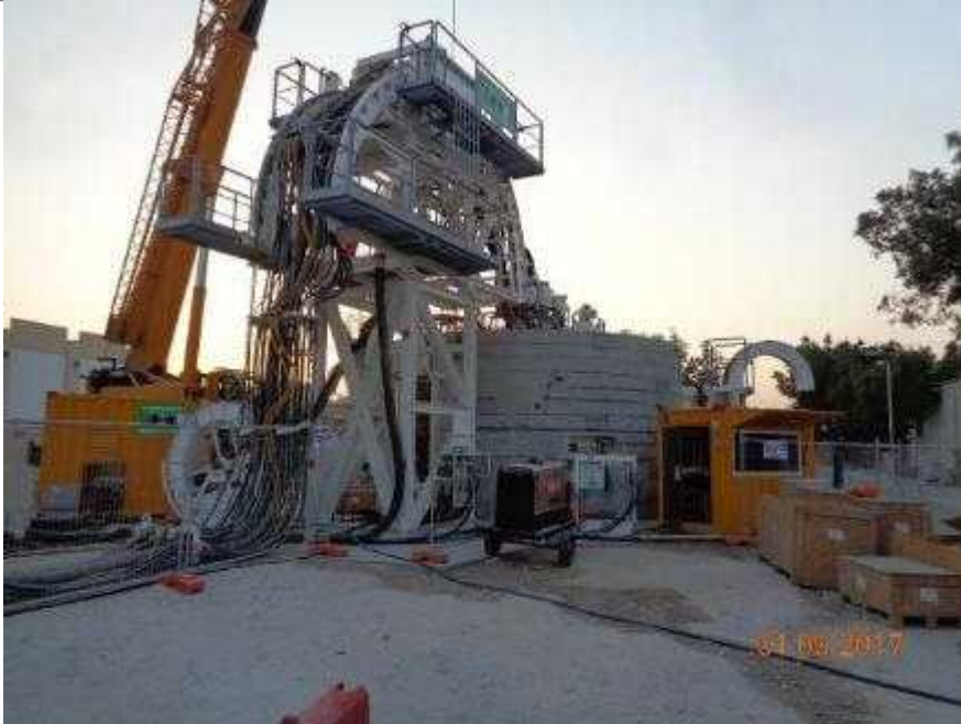
VSM Shaft Excavation Started
