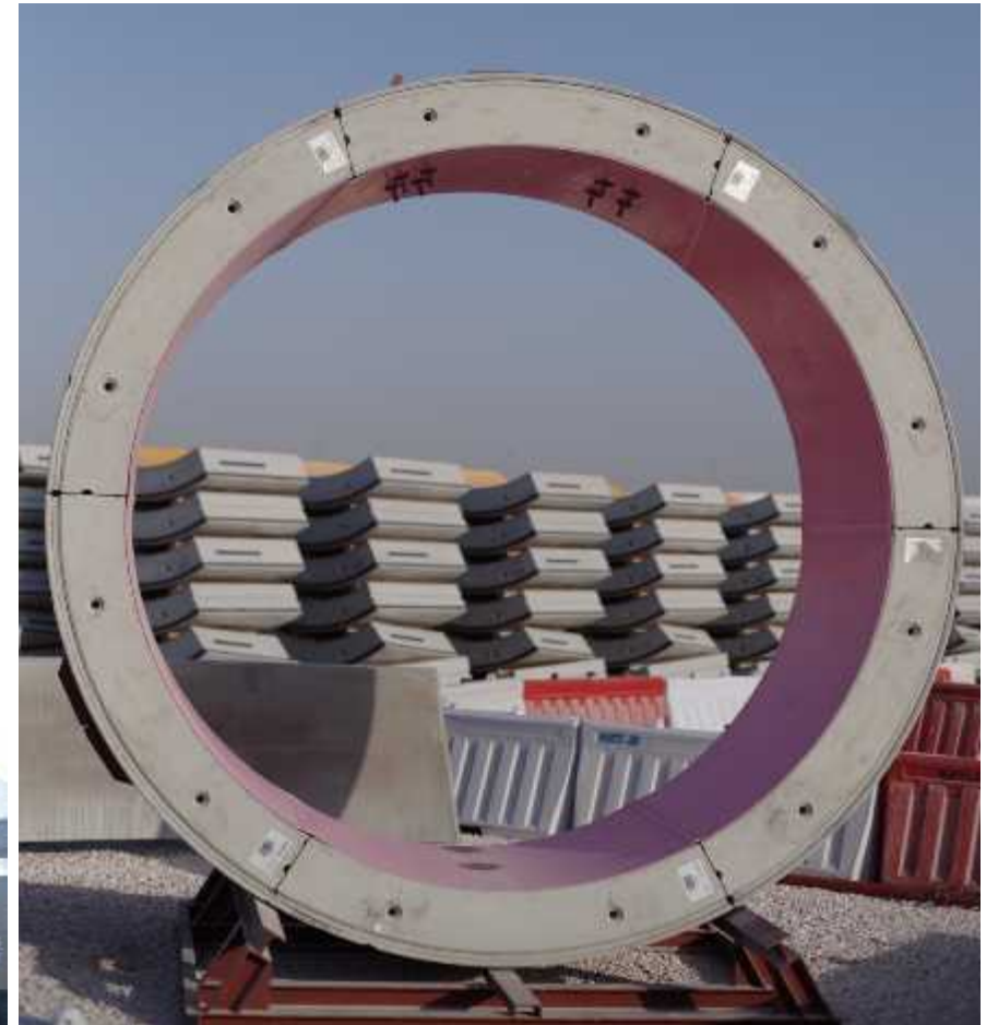
Typical 3m dia. Tunnel Ring – HDPE membrane installed and welded at the inner face
