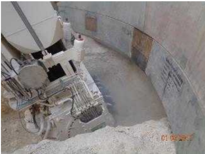
VSM Shaft Excavation Started
