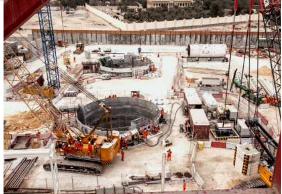
Main Tunnel Drive Shafts Completed
