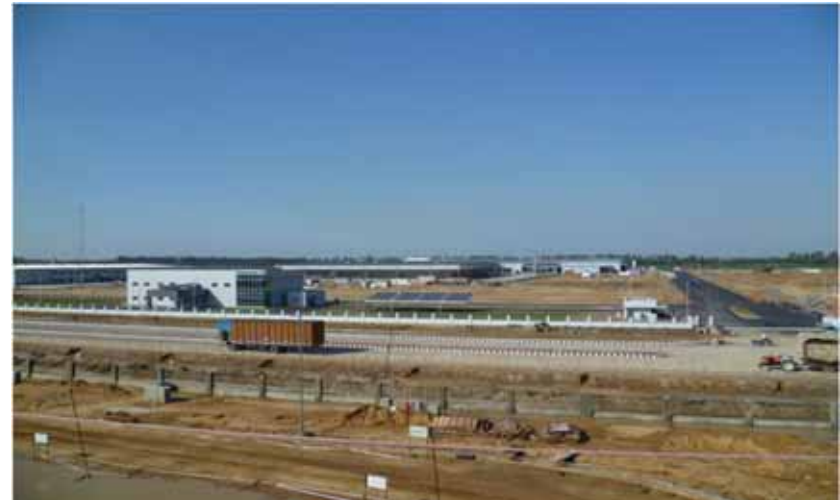
Site at the Time of Completion
