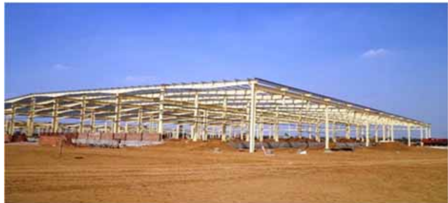
Steel Frame Ordered in Advance
