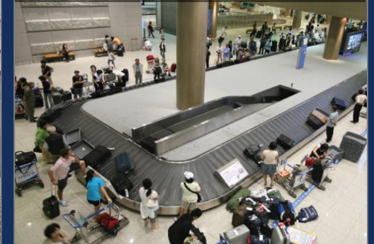
Baggage Handling System
