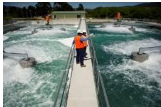
Cat D – NSW Public Works
