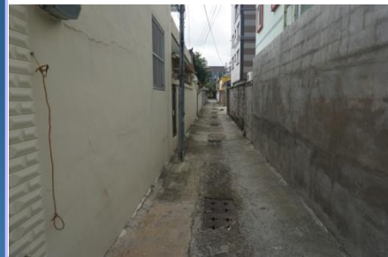
Deterioration of Residential Environment
