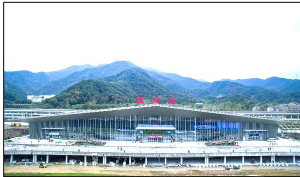
富阳站全景图 Full view of Fuyang Station
