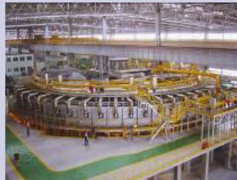
Heat Treatment Furnaces
