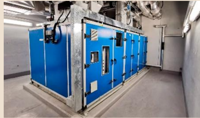
Integrated Air Handling Unit
